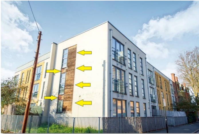
Maitland Road Elevation, 10 Maitland Road
