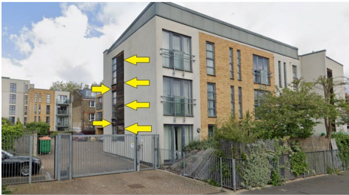
Maitland Road Elevation, 10 Maitland Road
