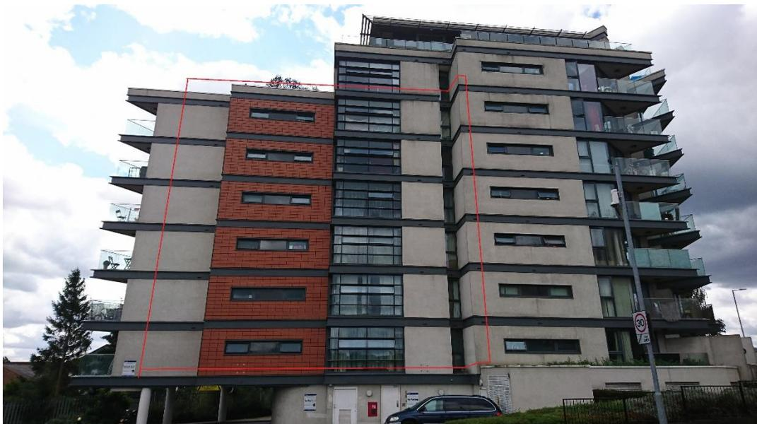
We have commissioned Philip Pank Partnership, an experienced building surveying practice to lead these investigations. They will be assisted by our contractor AD Construction Group to provide the scaffolding and labour to remove and re-fix the cladding finishes.
